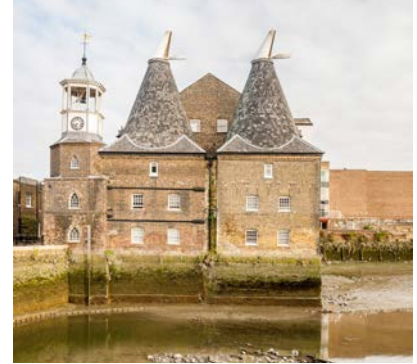
The Listed Mill Buildings opposite the site
