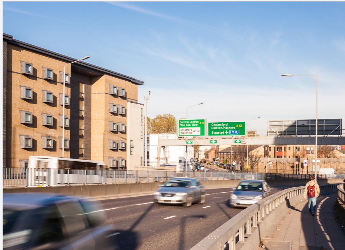
B View on A12 from the Southwestern corner of the development site
