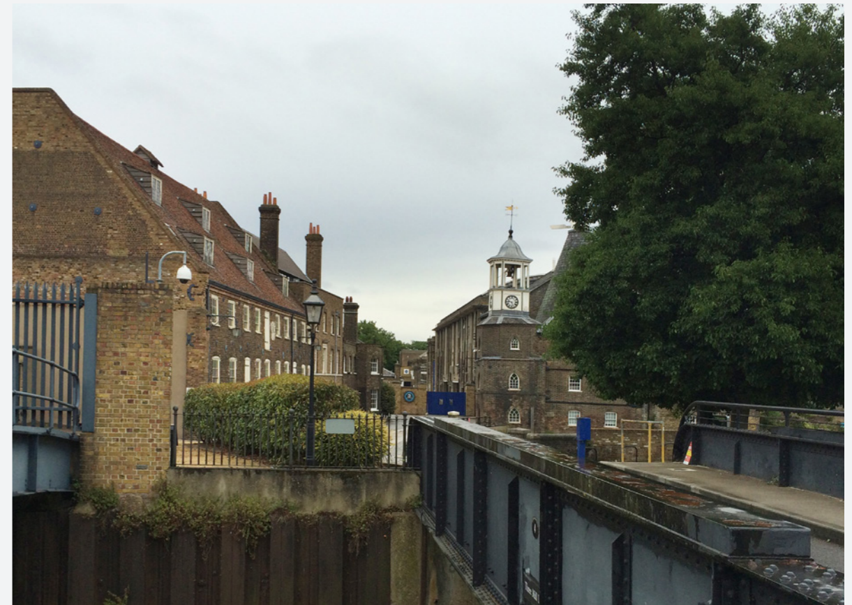
D View from the existing bridge towards the historic Three Mills
