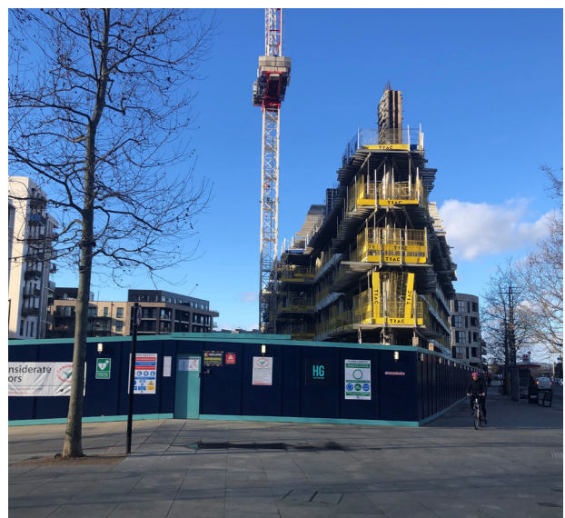
Image: East Village N05 progress
