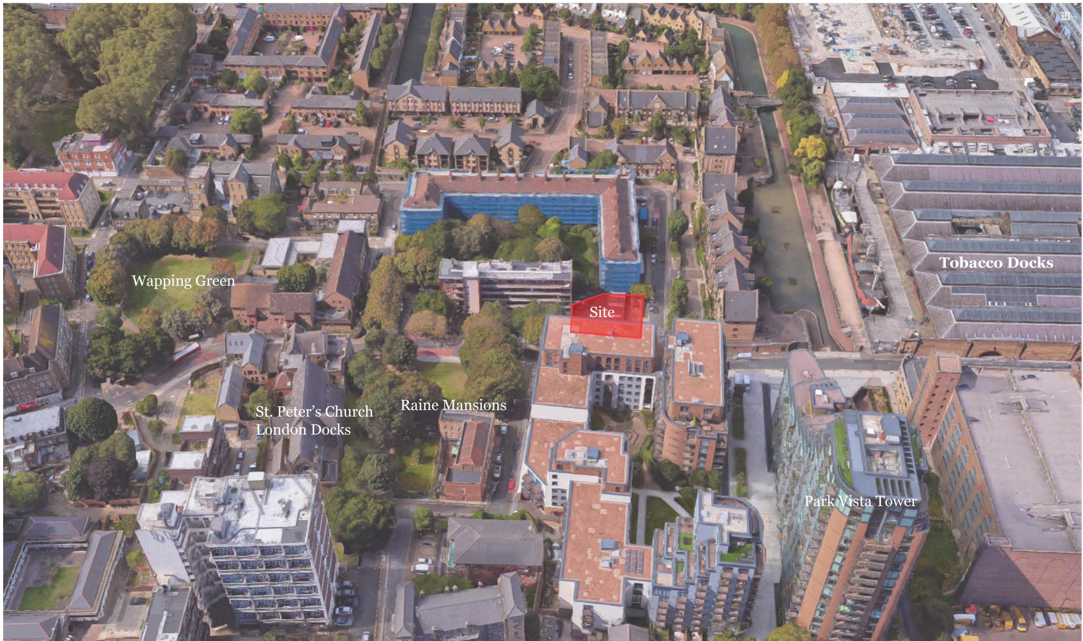
Aerial view of site (courtesy of google maps)
