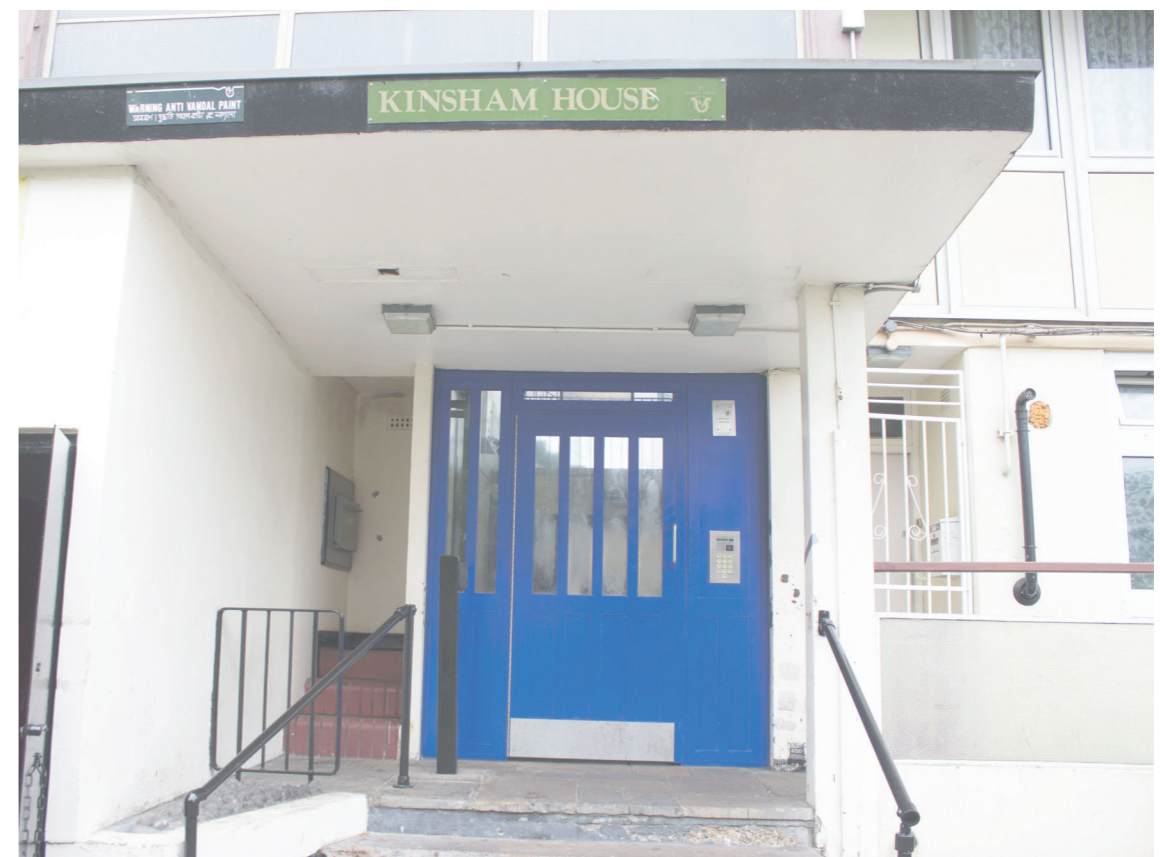
Existing main entrance
