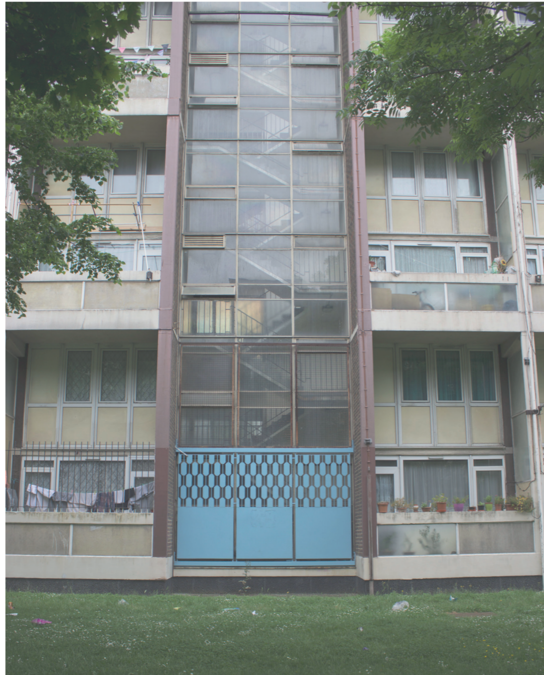
Existing circulation core
