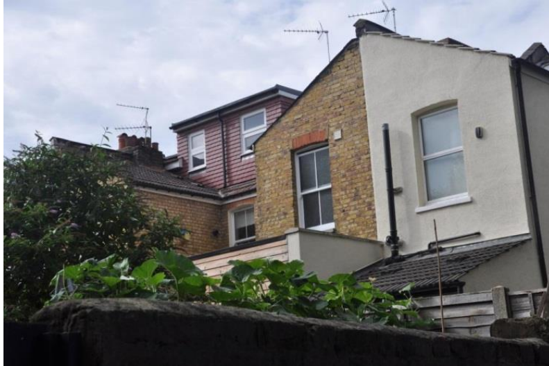
Two storey full height original extensions and single storey lean-to roofs (above).
