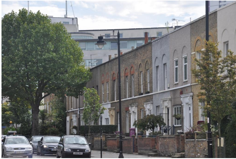
Fairfield Road (above): London (or Butterfly) roofs concealed from the street behind a continuous parapet. Chimney pots are the only historic element to break the skyline formed by the parapet.
