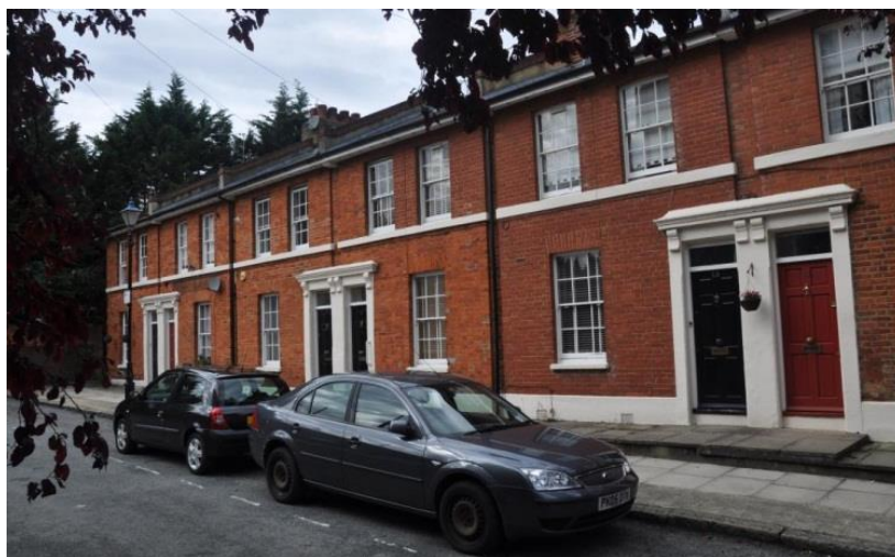
Hartfield Terrace (above): Gentle double pitched roof (with hipped ends): The roof unifies the terrace. A straightforward type of roof it is relatively rare in large parts of the Borough.
