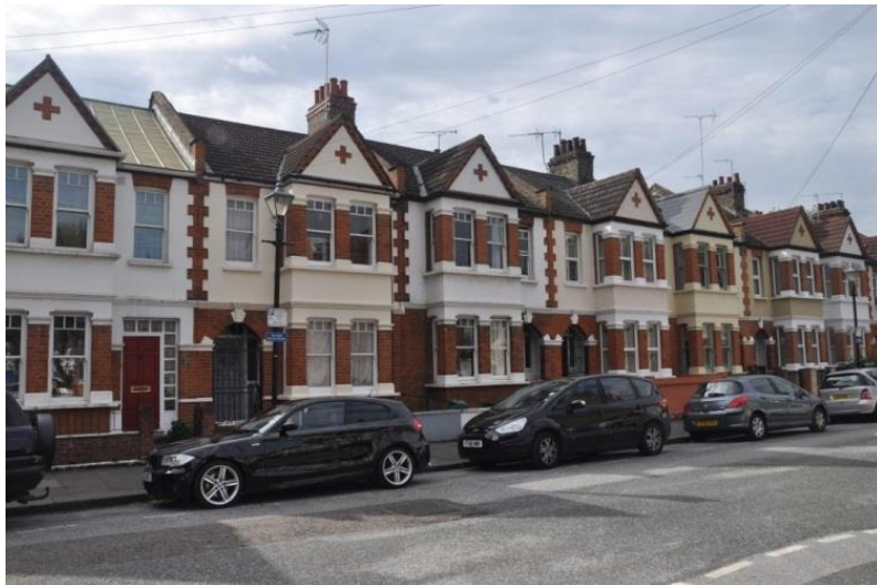
Steeper Double pitch roof with gabled ends and front gable over projecting bay (above): This type of main roof is very common in many parts of London but is rare in Tower Hamlets because of the age of much of the housing stock within the borough. The party walls project through the slope of the roof. Lots of these roofs on Wrexham Road and Ridgdale Street have been altered by the addition of a large dormer to the rear. This is less visible from the public realm.
