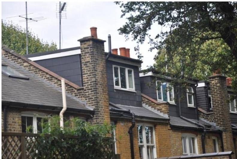
Ridgdale Street (above): Rear Box Dormers added to double pitch roofs
