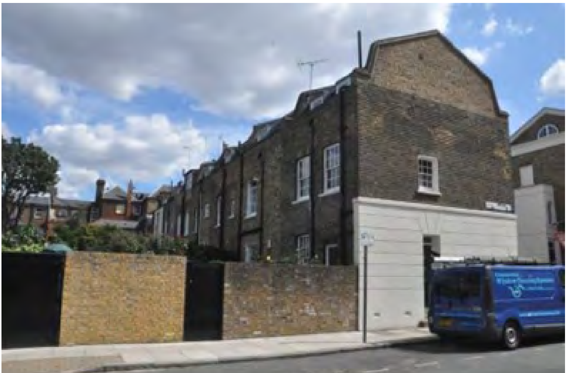
Tredegar Terrace (above): This terrace is flat backed, and this is an important part of the character of these earlier terraces. Those terraces around Tredegar Square itself have flat backs, with services being accommodated within the basement.
