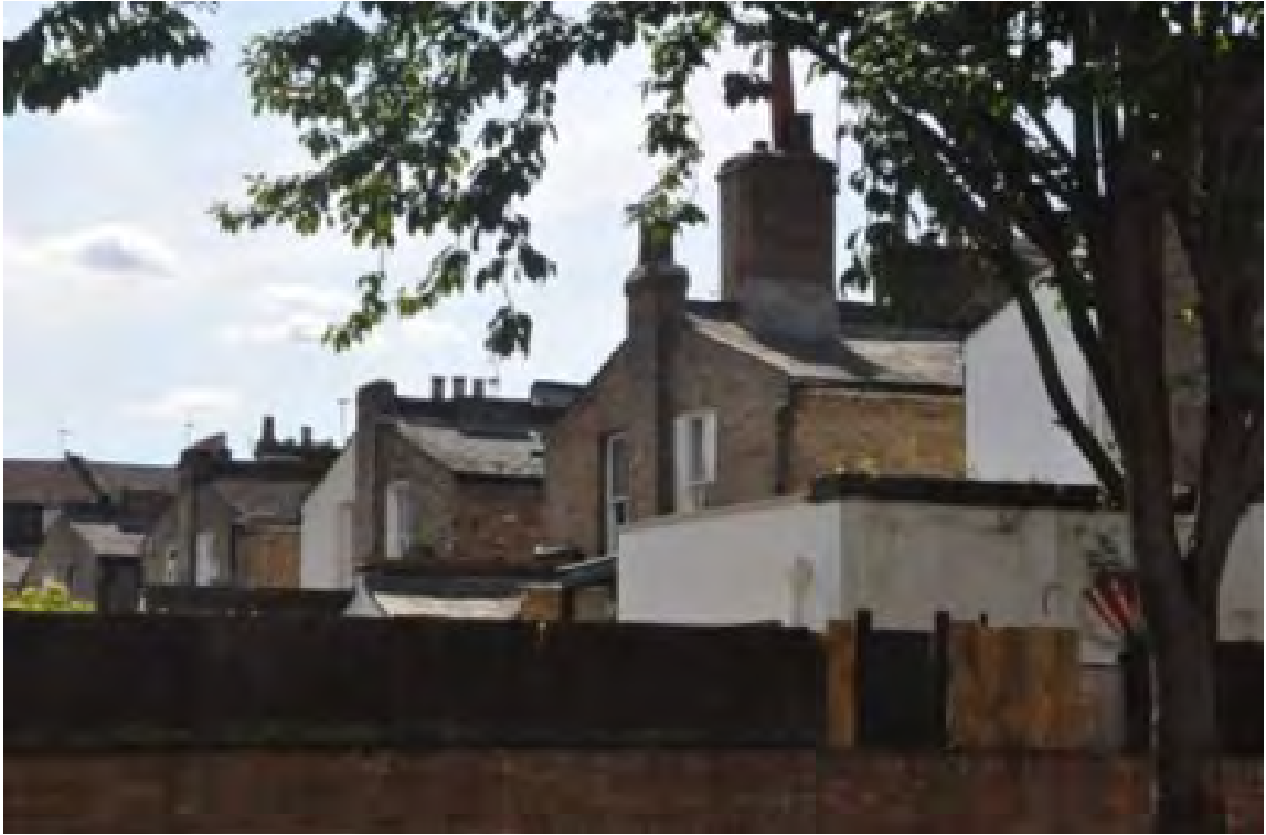
Rear of Alloway Road (above): Paired two storey projections with tall part immediately adjacent to main body of house and lower section beyond.
