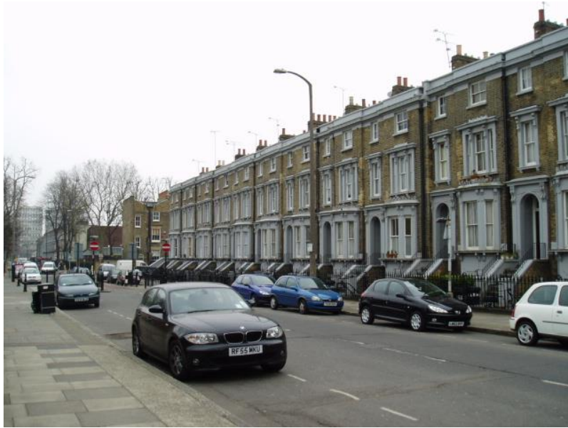
Bonner Road (above): the moulded cornice emphasises the strong parapet line.
