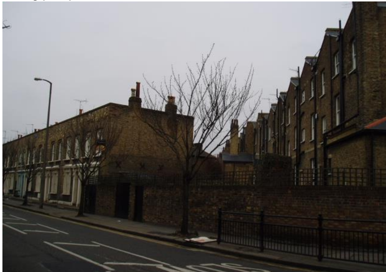
London (or Butterfly) roof (above): note the strong parapet to Old Ford Road and the rising and falling gables on the rear elevation of the houses to the right. Chimney pots are the only historic element to break the strong silhouette created by the parapet. This consistency is important to the character and appearance of the Conservation Area. The parapet is omitted from the rear elevation of houses with London roofs exposing the distinctive pattern of gables and valleys to view.
