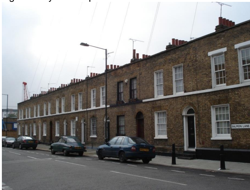
Salmon Lane (above): The London (or Butterfly) roof, concealed from the street behind a continuous parapet is highly characteristic of large parts of the York Square Conservation Area. In this particular example the parapet line is broken by chimney pots, this creates a strong and distinctive silhouette important to the character and appearance of the Conservation Area.
