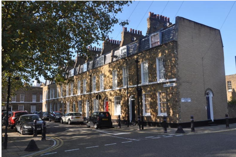
Original mansards facing the open space on York Square (above): the one at either end is hipped, it is this which allows the gable to have a straight top.
