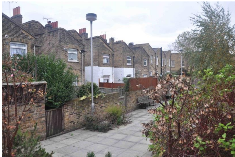
Rear of houses on Barnes Street showing two storey rear extensions with mono pitch roofs (above).
