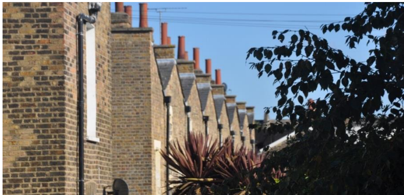
Rear of Matlock Street from the Burial Ground (above).
