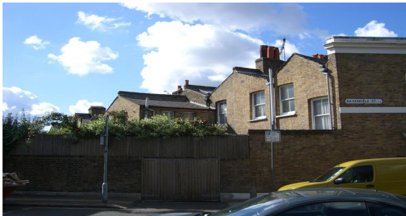
London (or Butterfly) roof (above): rear elevation of Barnet Grove from Baxendale Street. The parapet is omitted from the rear elevation of houses with London roofs, exposing the distinctive pattern of gables and valleys to view.
