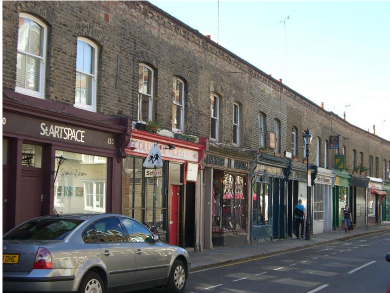
London (or Butterfly) roof - street elevations in Wimbolt Street and Columbia Road (above): This type of roof, concealed from the street behind a continuous parapet is highly characteristic of large parts of the Jesus Hospital Conservation Area. This consistency is important to the character and appearance of the conservation area.
