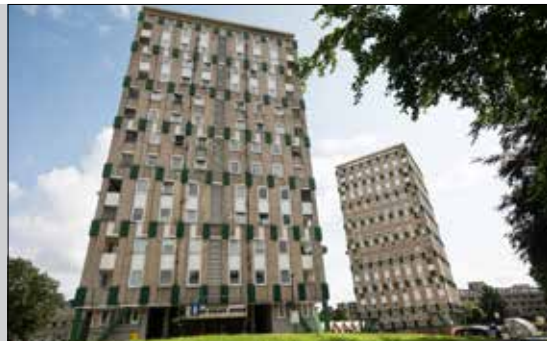
(13) Lubetkin's towers in the Cranbrook Estate
