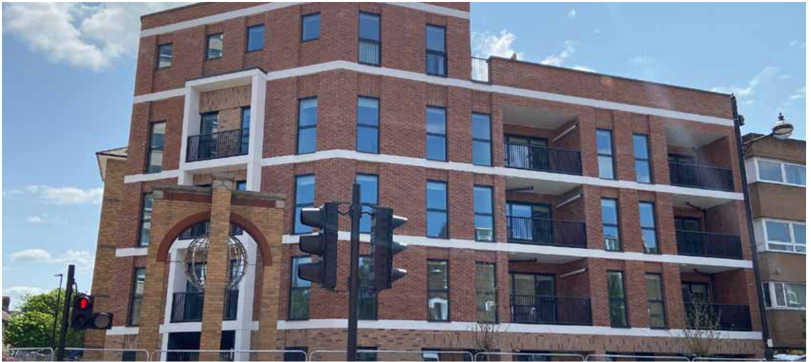
Sufia Kamal House, which is one of the new housing blocks nearing completion
