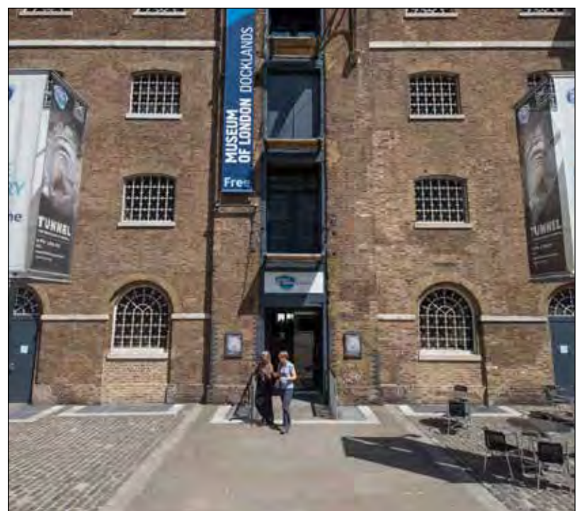
The museum building was originally a 19th century quayside warehouse
