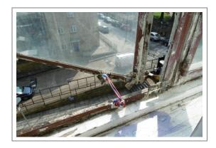
Deteriorated external window cills
