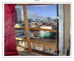
Metal window inappropriately repaired with battens
