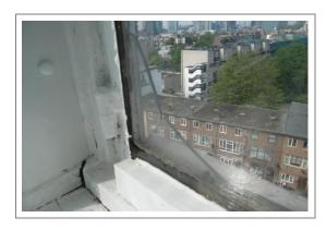
Falling internal cills strutted with battens
