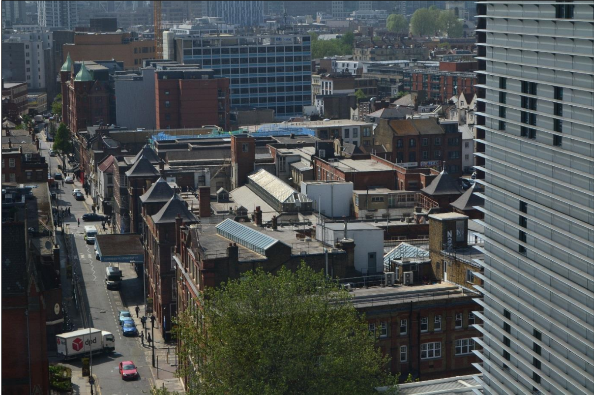
Photograph 5 – Looking West along Stepney Way from Hospital
