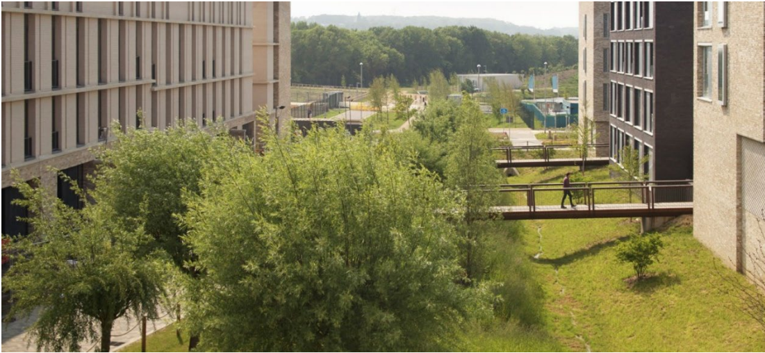
Plate 12: North West Cambridge Integrated SuDS feature. Source: AECOM (2019)
