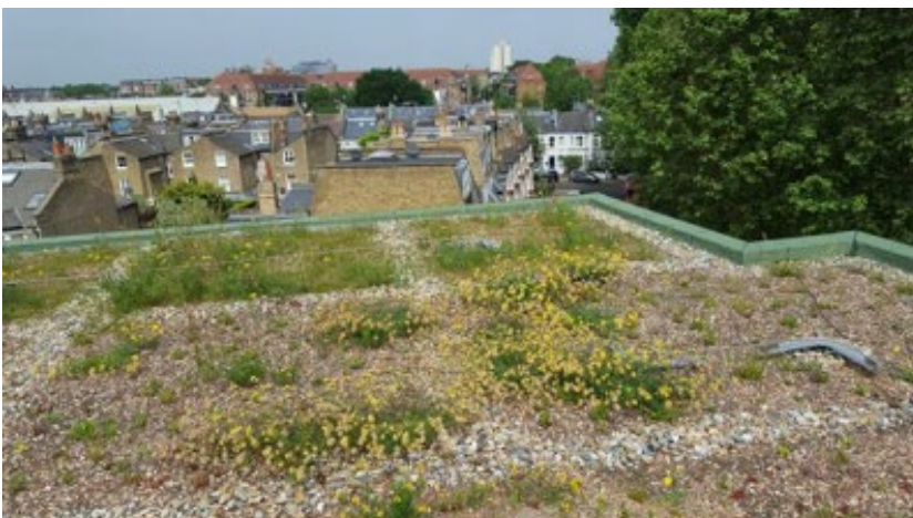
Plate 10: Richard Knight biodiverse extensive green roof
