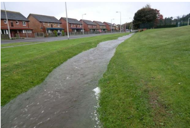
Figure E.36: Example of a swale channel
