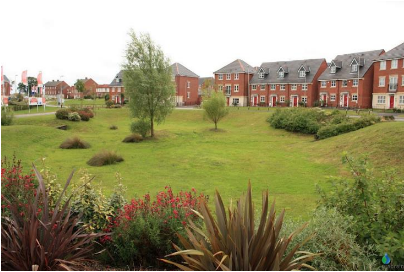
Figure E.37: Example of a detention basin
