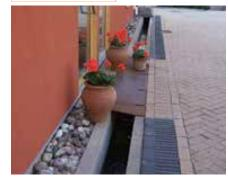
Figure 6-12 Example of rills that convey runoff along the surface. SuDS Manual C753.
