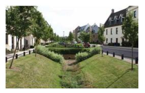
Figure 6-4 Example of swale providing a vegetated corridor. SuDS Manual C753.
