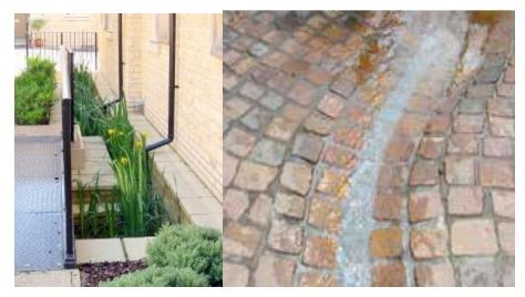
Figure 6-8 Example of drainage channels and rills. SuDS Manual C753.
