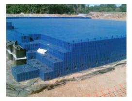
Figure 6-11 Example of geocellular units being constructed. SuDS Manual C753.
