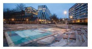
Figure 6-21 Example of urban hard surfaced off-line detention basin. SuDS Manual C753.
