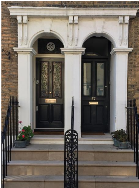
The paired doorways with painted stucco surrounds are characteristic of the area
