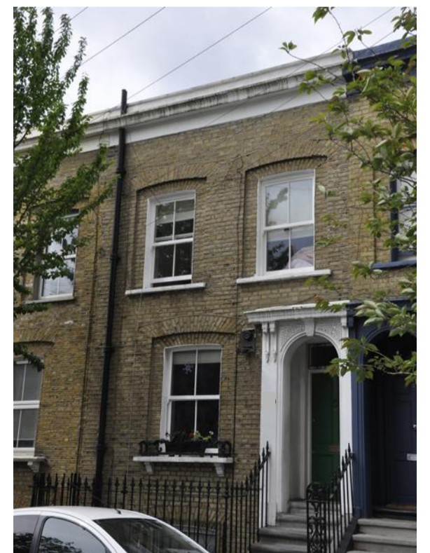
Driffield Road cornice penetrated by pipework
