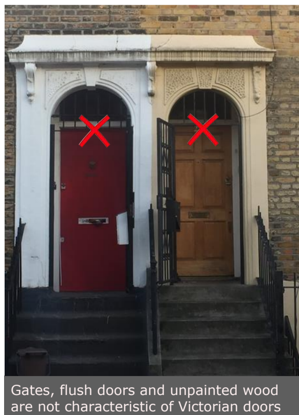
Bringing forward the door reduces the depth of modelling on the facade
