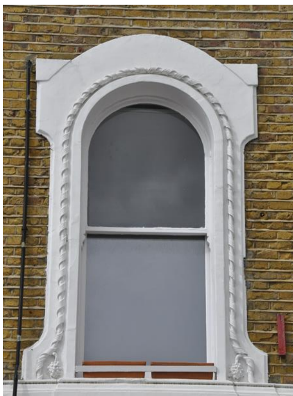
Hewlett Road first floor window with characterful rope moulding with grapes
