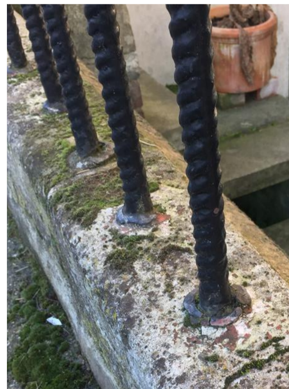
Bars lead caulked into stone base
