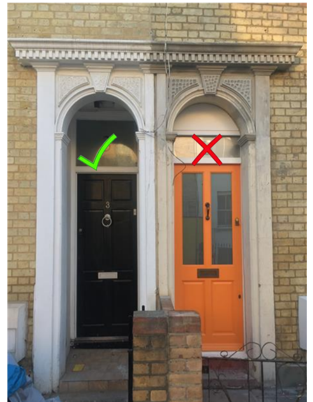
Bringing the door forwards in the opening reduces the modulation on the street
