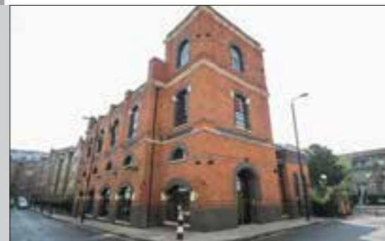
(3-4) Hooper Street Pump House
