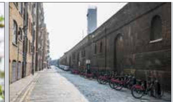
(6) Pennington Street warehouses
