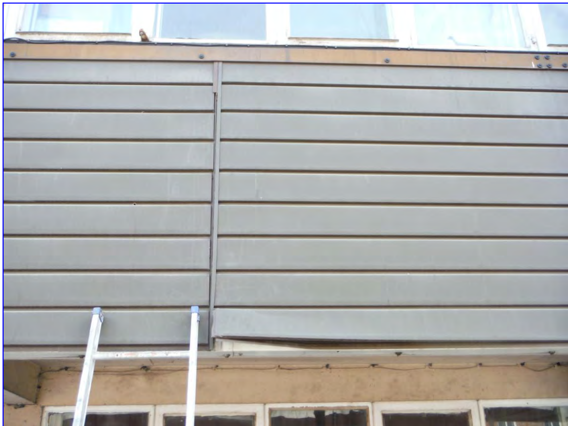
Photograph 19: General view showing typical metal cladding (on Lister House).
