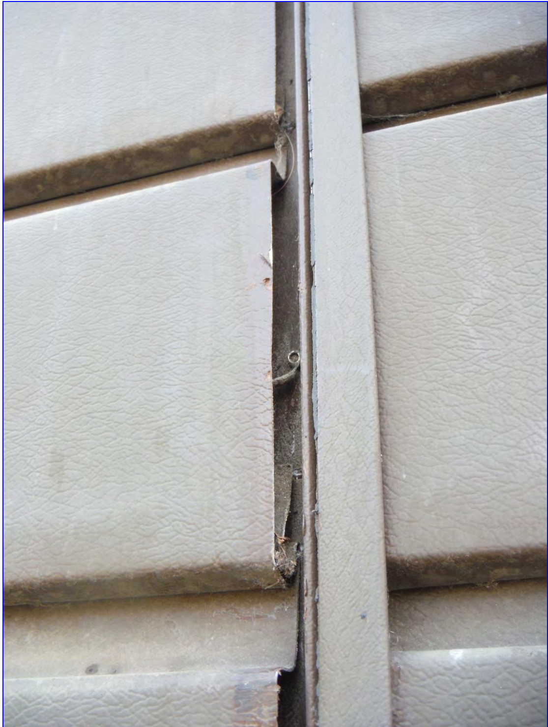
Photograph 24: View showing typical metal cladding profile externally.
