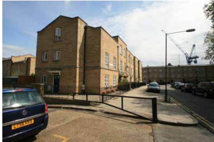
1. Looking East along Lomas Street. Existing 2&3 storey residential perimeter to Vallance Gardens and service road to Lister & Treves House.
