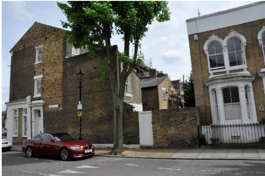
Rear extensions viewed from Arbery Road
