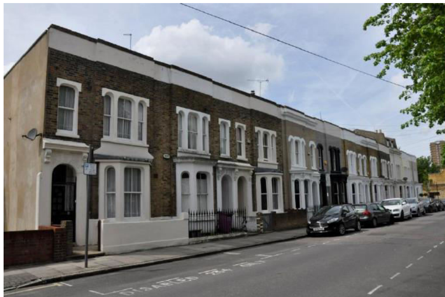
Terrace on Selwyn Road; the houses have canted bay windows but only three houses retain their cornice.
