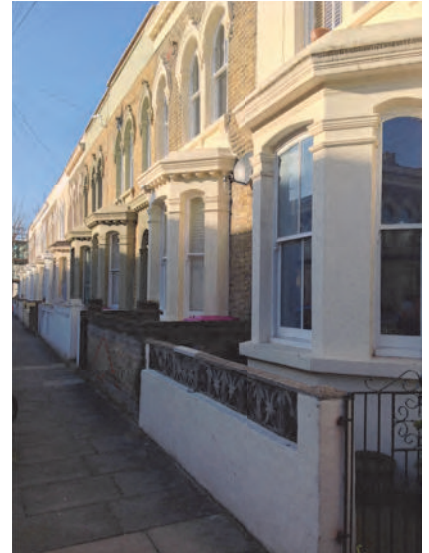
Strahan Road- loss of character
