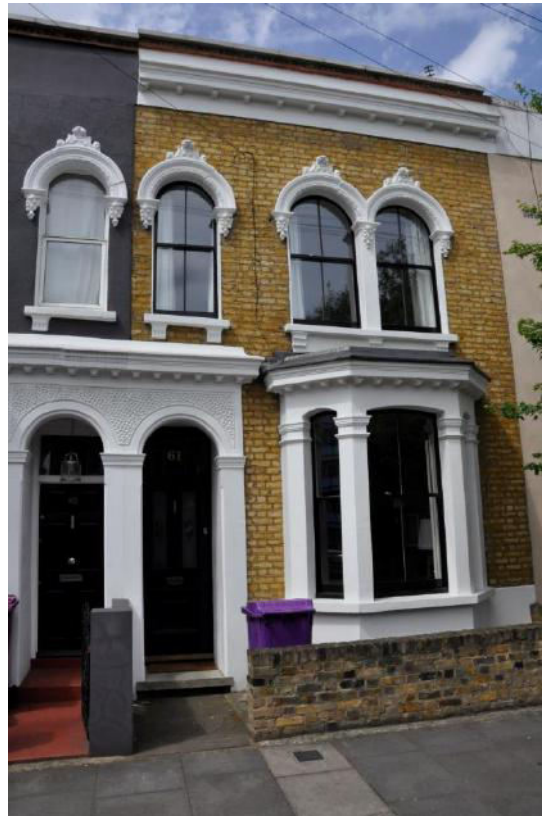
Strahan Road (with original cornice intact).
