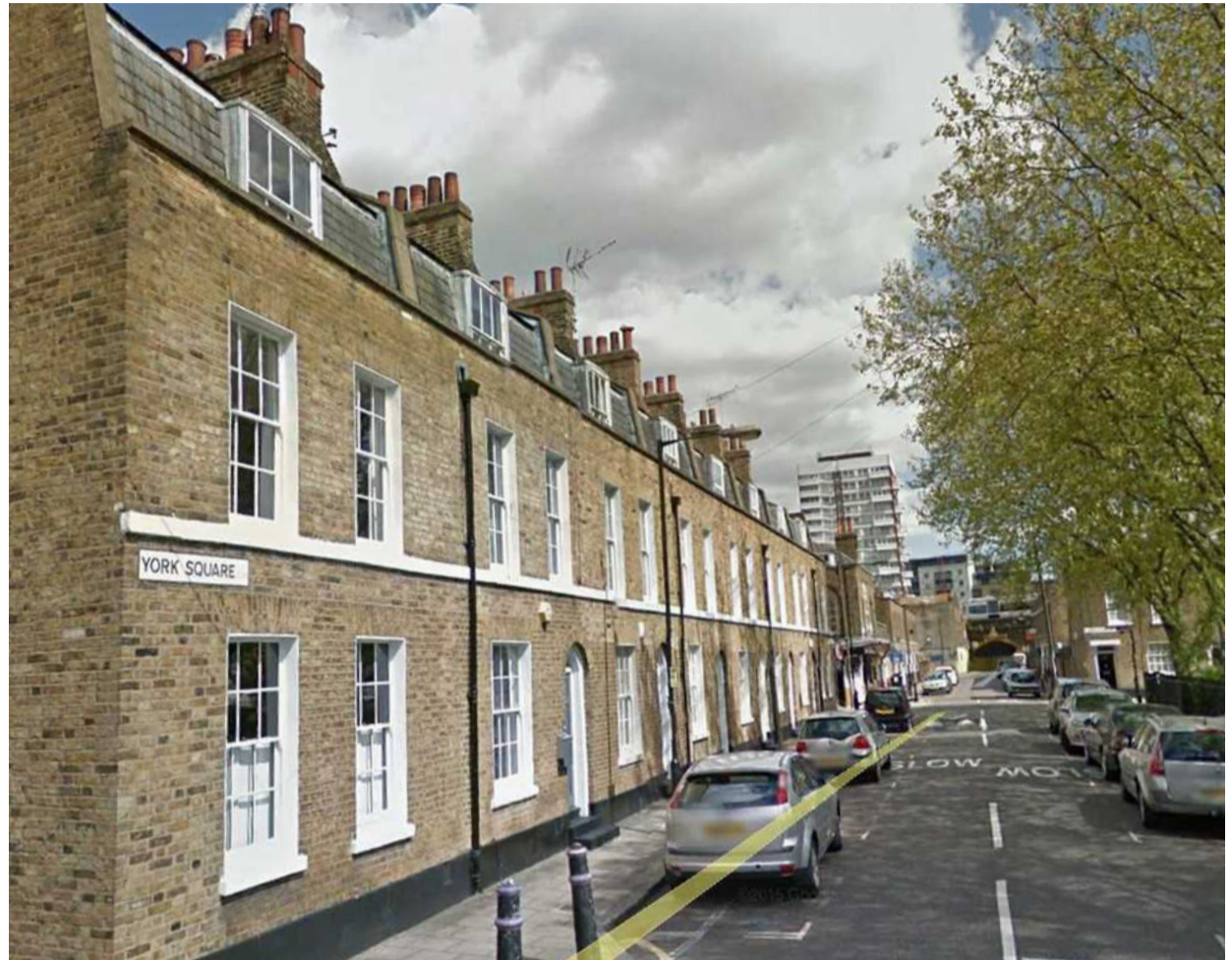
A unified approach to design was adopted when mansard roof extensions were added to York Square E14
