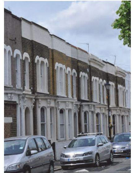
Loss of cornices reduces the architectural character
