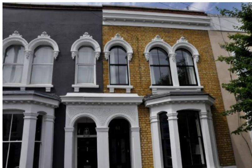
Detail of round-headed paired window openings with stucco surrounds and foliate embellishment and reticulated stucco around the door.
