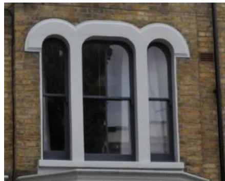
Detail showing tripartite round-headed window openings with sash windows.
