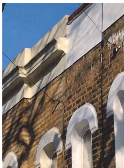
Typical curved stucco moulding over first floor windows in Medway Conservation Area
