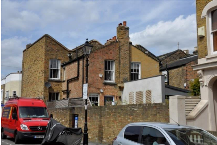
London Roofs visible along Medway Road.
